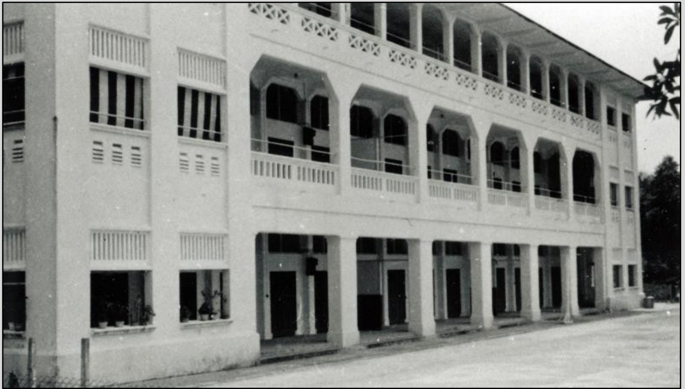
The 'cookhouse' block and 84's barrack accommodation
